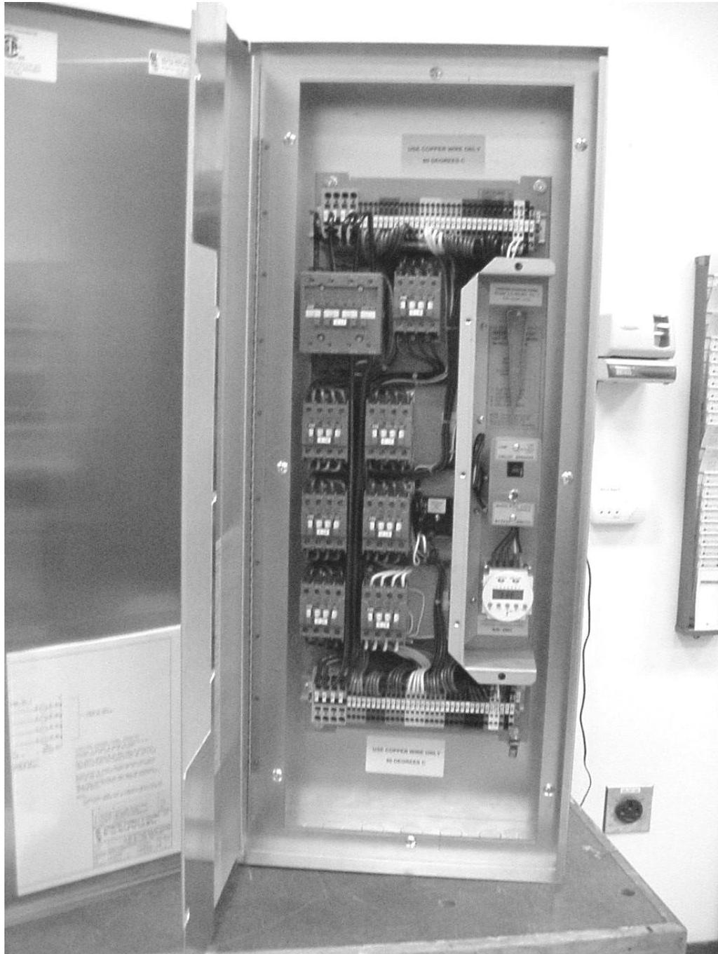
**OVERALL VIEW LC PANEL SHOWING SUB PLATE WITH CONTACTORS**
