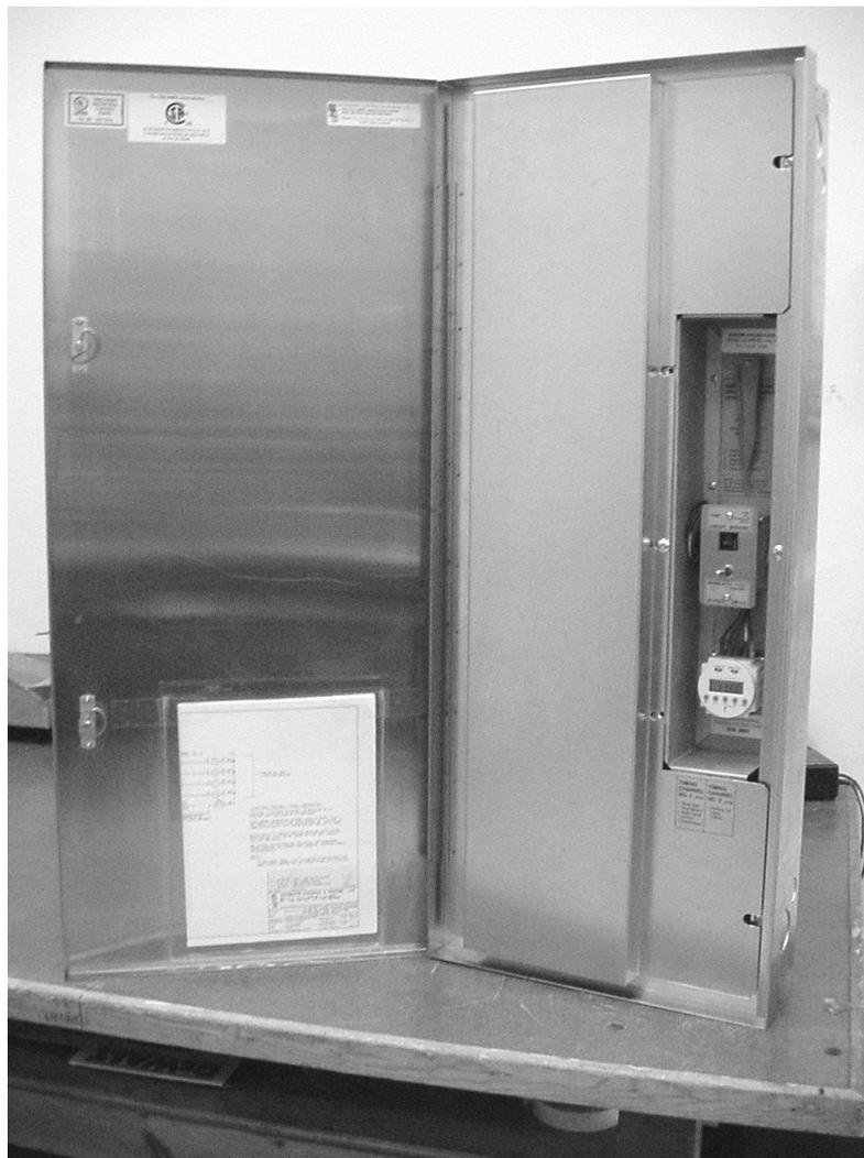
**MODEL LC LIGHTING CONTROL PANEL WITH MAIN DOOR OPEN**
