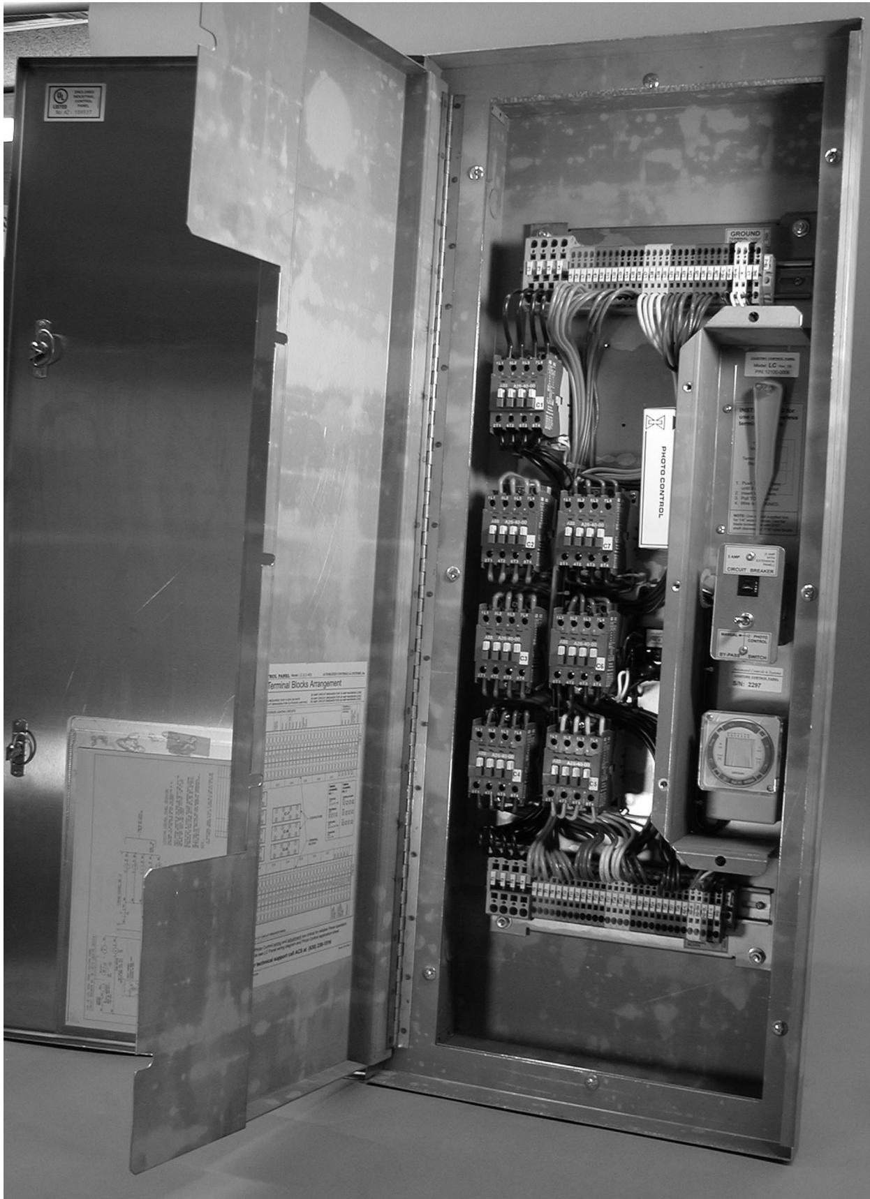
OVERALL VIEW OF LC PANEL SHOWING SUB PLATE WITH CONTACTORS
